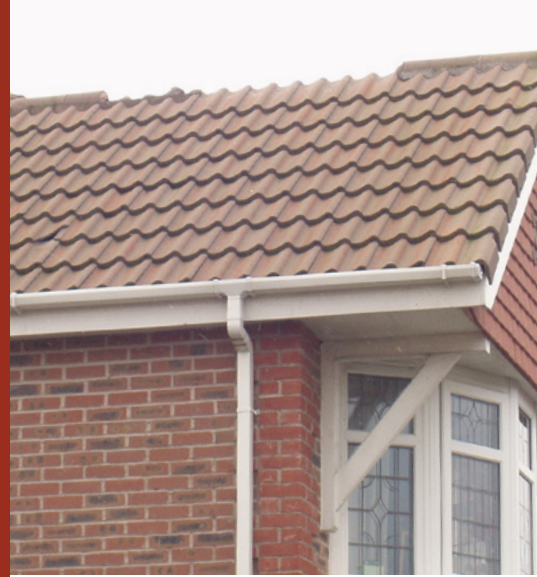
Typical storm damage to hip due to reliance on mortar alone.
